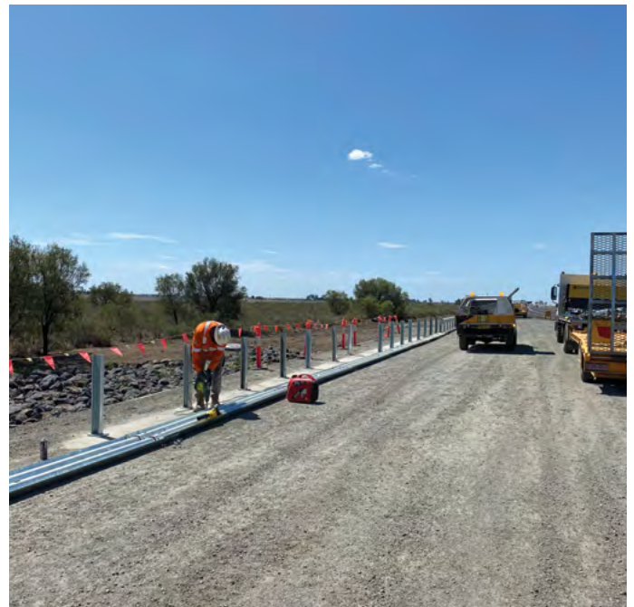
Installing new guard rail in Section 5 north of Clarks Gully
