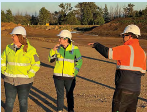
NSW Minister for Regional Transport and Roads Jenny Aitchison inspecting the rest area site with the project team in July
