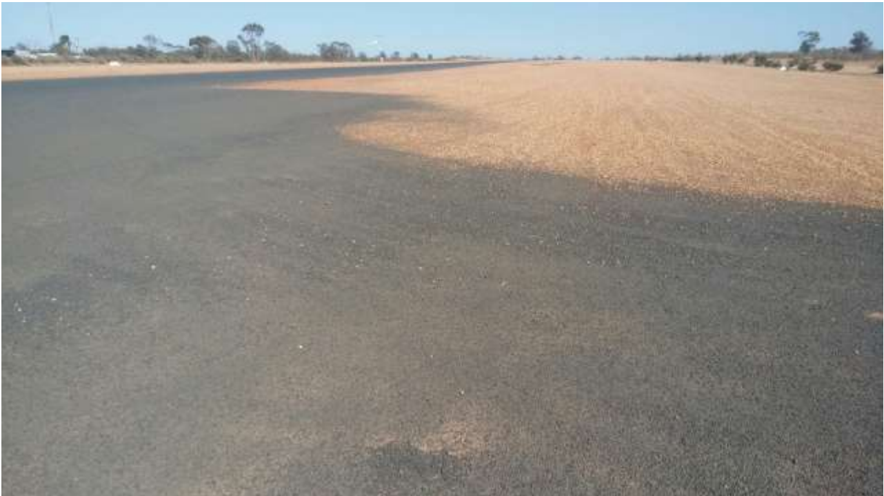
Taxiway to Parking Apron
